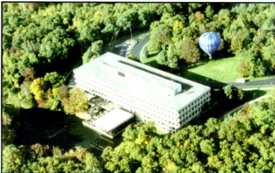
Union Camp World Headquarters, Wayne, N.J. Chris James Landscaping provides year-round service in snow removal and Landscape management
